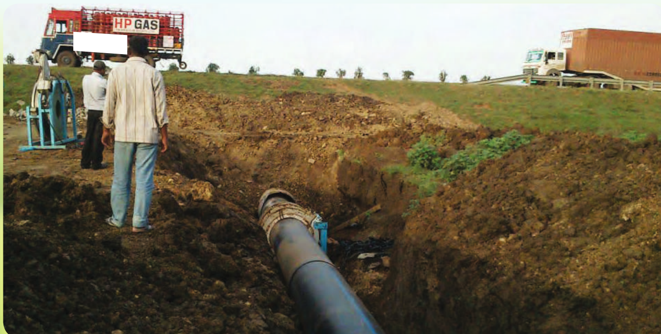
Use of HDPE Strong and Durable pipe for Highway Crossing
